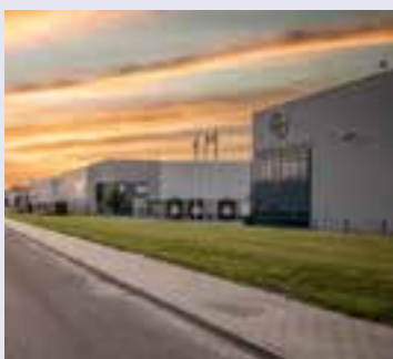
P3 Blonie: Polish warehouse complex was part of P3 buy
